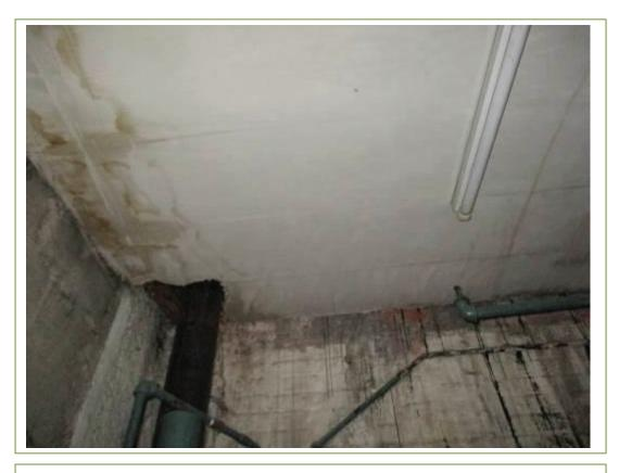
Plasterboard ceilings in sprinkler room. No ACM's detected
